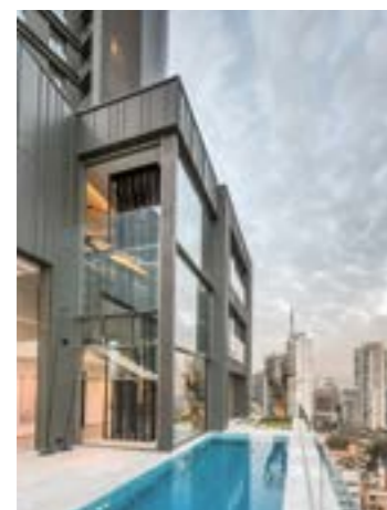
Project in Lebanon
